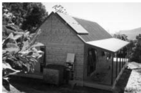
A typical RAPS system with generation equipment
